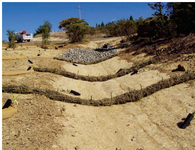
Install wattles or erosion control mats to reduce soil erosion.
