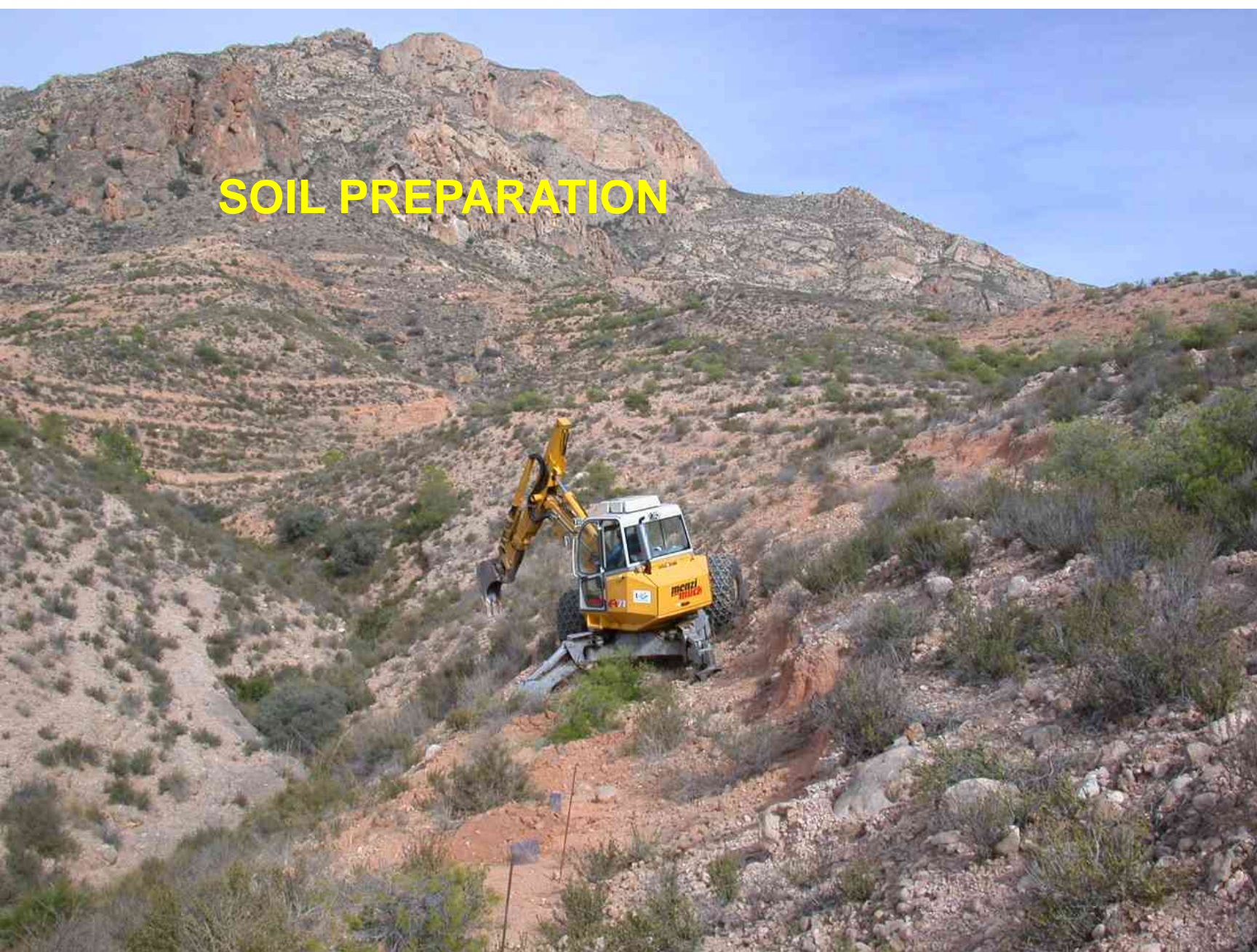
Mechanical hole with backhoe Spider
