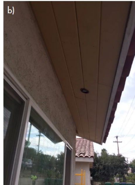
Figure 6. Images of a) open eave design that may allow ember penetration into the structure more readily than b) closed eave design that has been significantly associated with structure survival in California wildfires.
