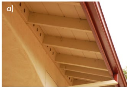
Figure 6. Images of a) open eave design that may allow ember penetration into the structure more readily than b) closed eave design that has been significantly associated with structure survival in California wildfires.
