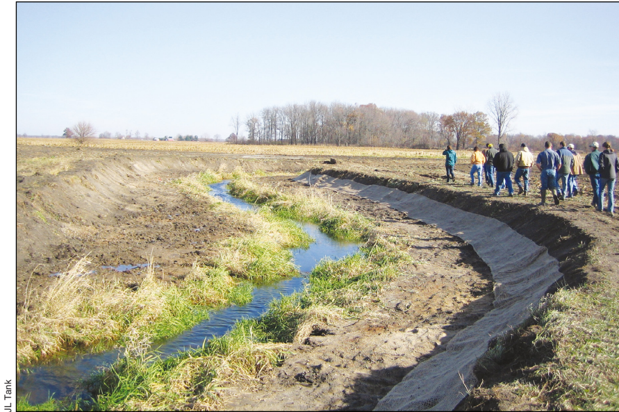
Figure 6. Resource managers and farmers tour a site following construction of inset floodplains designed to reduce nutrient and sediment export from the Shatto Ditch watershed in Indiana.
