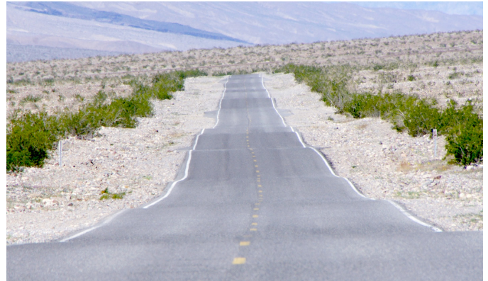
Figure 1. Scotty's Castle Road in the Mojave Desert crossing an alluvial fan, looking northwest. Enhanced creosote growth on the sidecast banks is evident.
