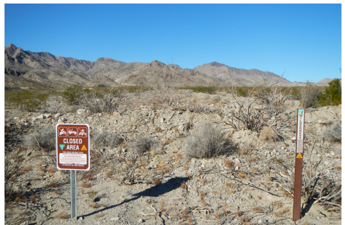
Figure 10. Vertical mulch structures, shown in the bottom right of the photo and in the center-right (to the left of the top of the wilderness sign), as part of restoration on a decommissioned road in the Dead Mountains Wilderness Area, eastern Mojave Desert, southeastern California. The vertical mulch was constructed from collecting dead branches of creosote bush and arranging them vertically in the soil to mimic structure of a creosote bush shrub (albeit without live foliage). Photo taken in November 2016 by S.R.Abella.
