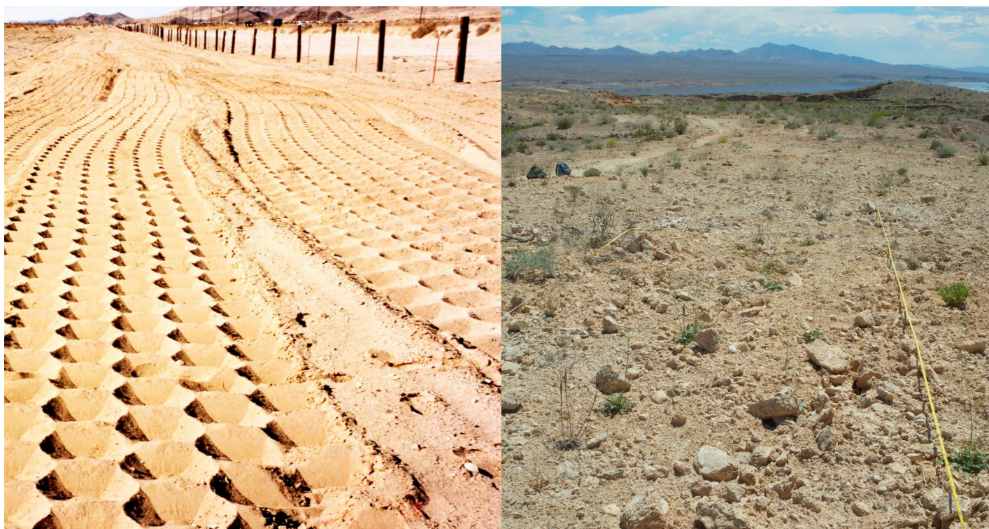
Figure 6. Examples of geomorphic restoration treatments for encouraging recovery on compacted and disturbed soils. Left photo: Imprinting intended to roughen the surface of compacted soil to deter erosion, retain nutrients and biotic resources, and create favorable conditions for native plant establishment (photo courtesy of D.A. Bainbridge). Right photo: Ripped road designed to de-compact soil and promote plant establishment on gypsum soil, Lake Mead National Recreation Area, eastern Mojave Desert, southern Nevada (S.R. Abella).
